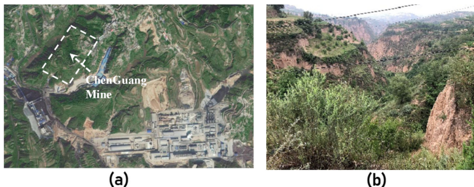
Fig. 4 Field site at Chenguang bauxite mine. (a) Geographical location map of the mine. (b) Image of the mine surface
