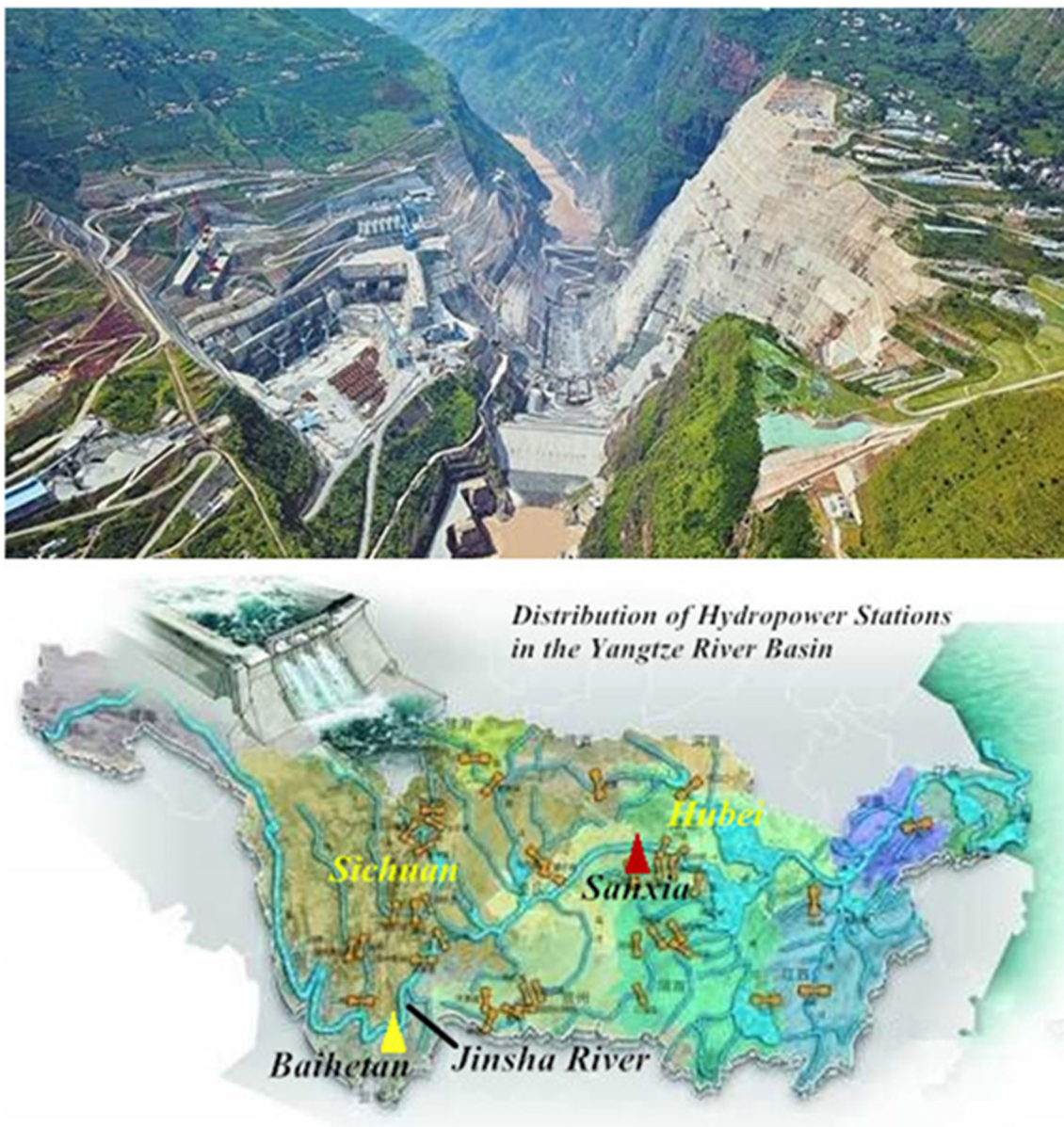
Fig. 1 View and location of Baihetan Hydropower Station
