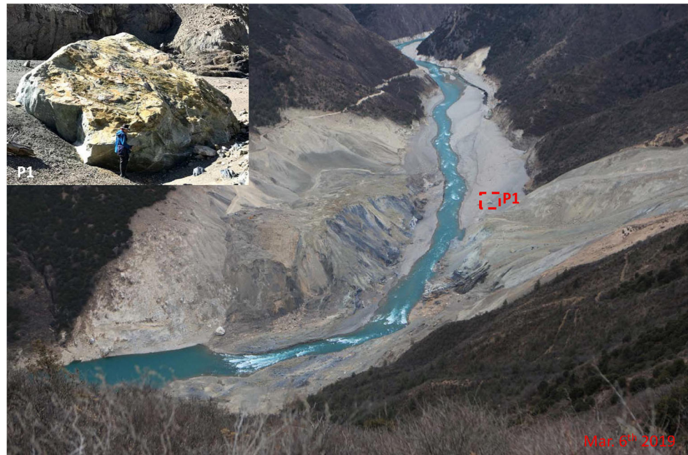
Fig. 17 Sluice channel after dam breaching of the “11.3” rockslide dam
