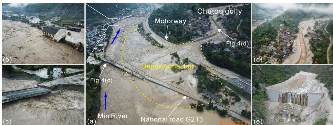
Fig. 4 Features of Chutou gully on Aug 20, 2019. a Panorama of depositional fan; b destroyed houses in downstream; c broken bridge; d affected village; e Gorged dam with debris flow materials, the location is showed in Fig. 2.
