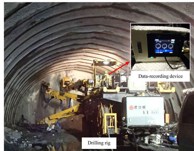
Fig. 2 Drilling rig and data-recording device
