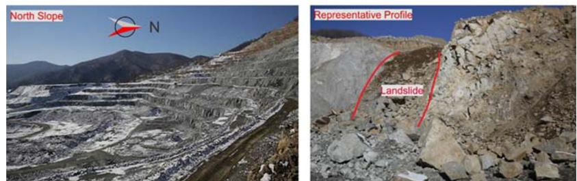
(b) Photograph of the research area and landslide
