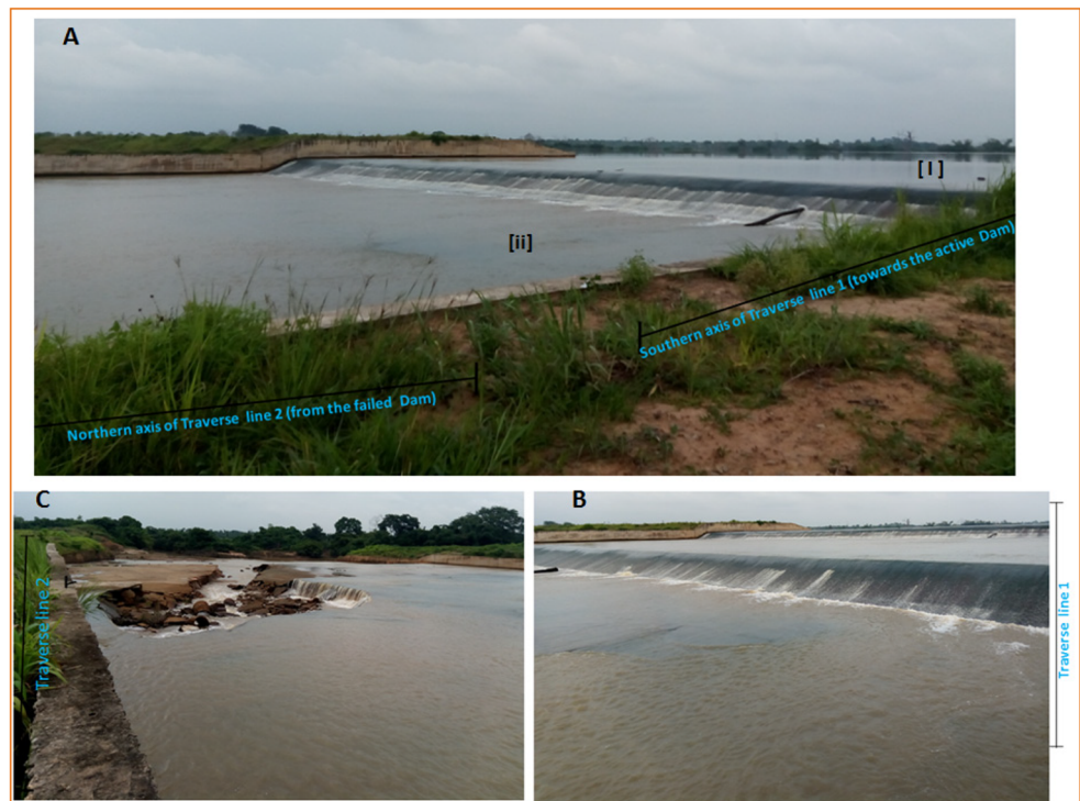
Fig. 1 The dammed water reservoirs. a Axis showing the downstream end of traverse line 1 between reservoir I (R-I) and reservoir II (R-II) and the upstream edge of traverse line 2. b Embankment demarcating reservoir I and II. c Downstream edge of traverse line 2 along the failing section of the dam by the tail water (R-III)
