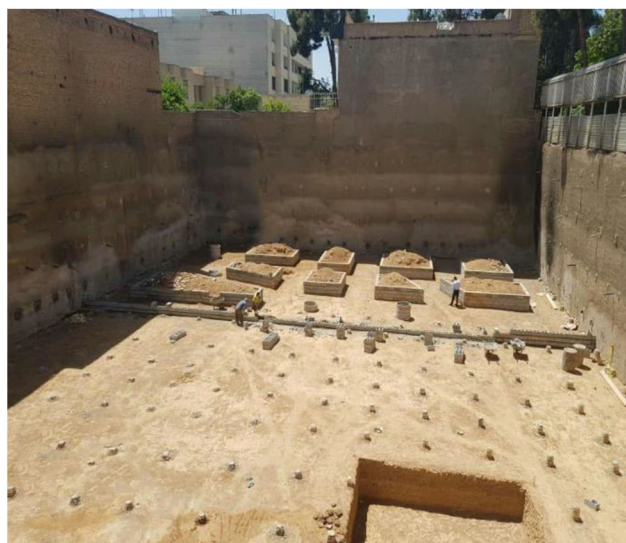
Fig. 24 Final view of soil nail wall and excavation
