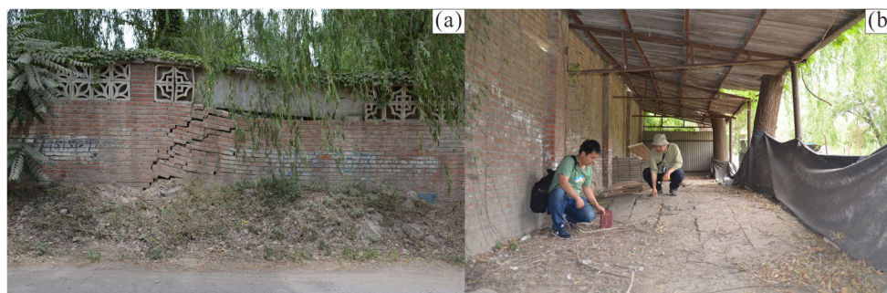
Fig. 14 Damages in the Wuyuan logistic park. Photos were taken on June 2, 2017. Location is shown in Fig. 10. Three-hundred-meter-long earth fissures trending N30 °~40 °E in the Wuyuan logistic park. Southeastern side has subsided 10~20 cm. Differential subsidence and
