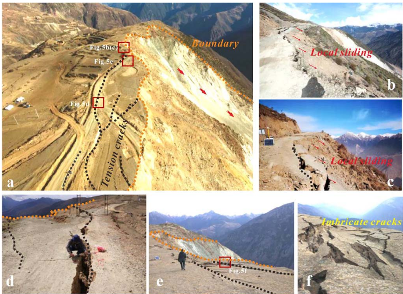
Fig. 8 Main characteristics of the W_block. (a) Location of the tension cracks after the second landslide; (b) local sliding after the first landslide; (c) local sliding after the second landslide; (d) crack opening width of up to 30–50 cm; (e) tension cracks developing; (f) imbricated cracks
