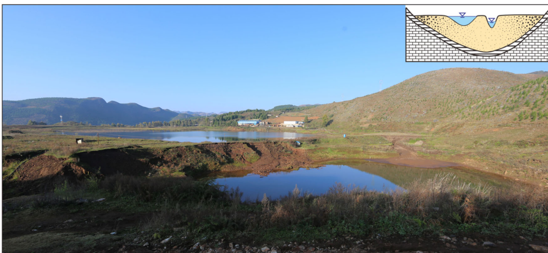
Fig. 11 Two adjacent ponds with different water tables within the AXZ tailings impoundment
