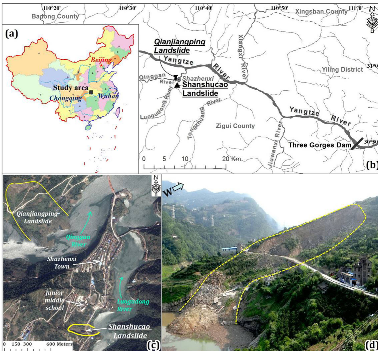
Fig. 1 Location and general overview of the Shanshucao landslide. a Location in China; b location in the Three Gorges Reservoir; c location in the town of Shazhenxi; and d general view of the southern rocky part of the failed landslide
