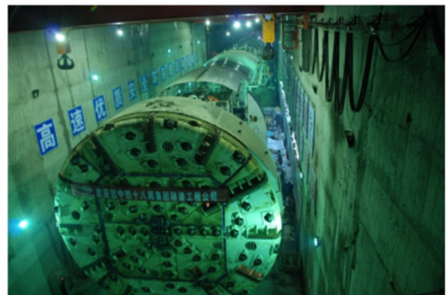
Fig. 2 An image of the tunnel boring machine manufactured by Robinson and Herrenknecht AG
