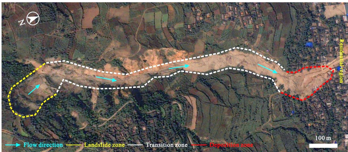
Fig. 13 Satellite picture of the Dagou landslide two months after its occurrence (modified from Google Earth)
