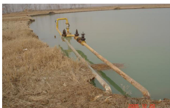
(a) The 2005 sinkhole
