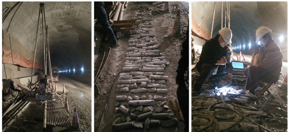
Fig. 15 Hydraulic fracturing test at Section K61 + 195 of Huangjiazhai Tunnel
