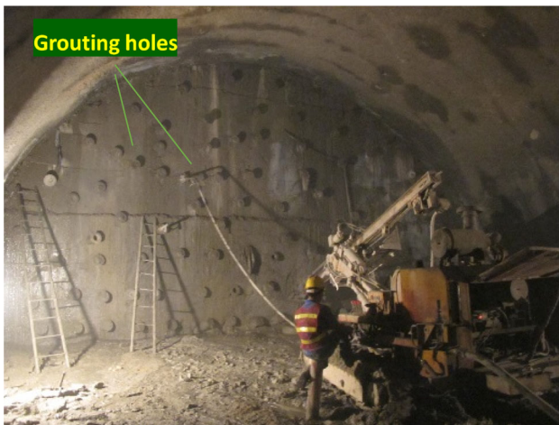
Fig. 12 Construction of curtain grouting
