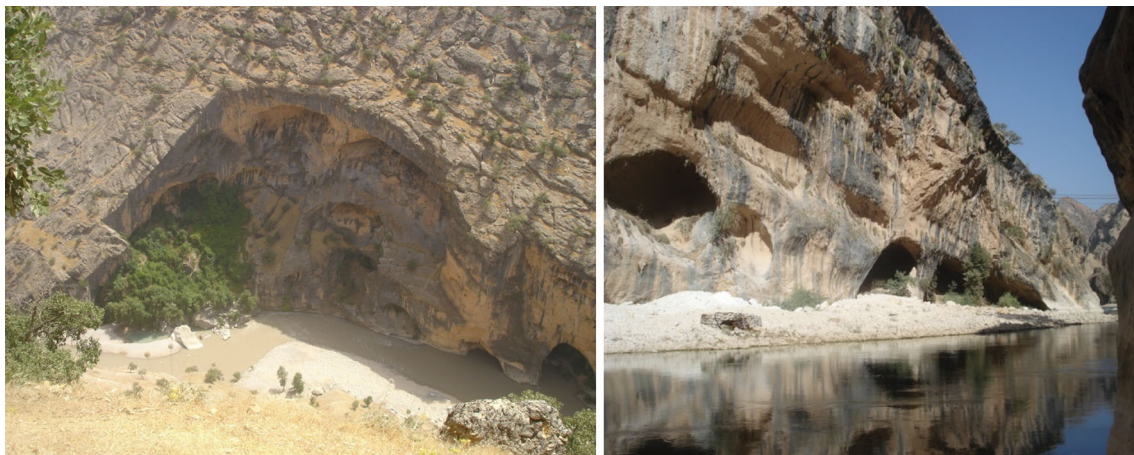
Fig. 3 Photographs of karstic features in the right abutment of Bazoft dam site
