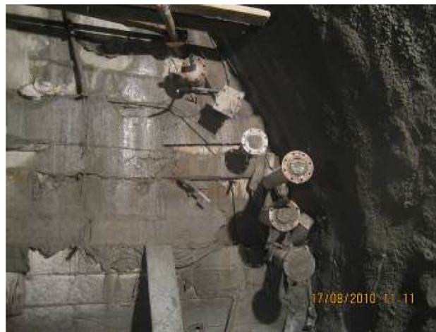
Fig. 11 Advanced long pipe-shed grouting
