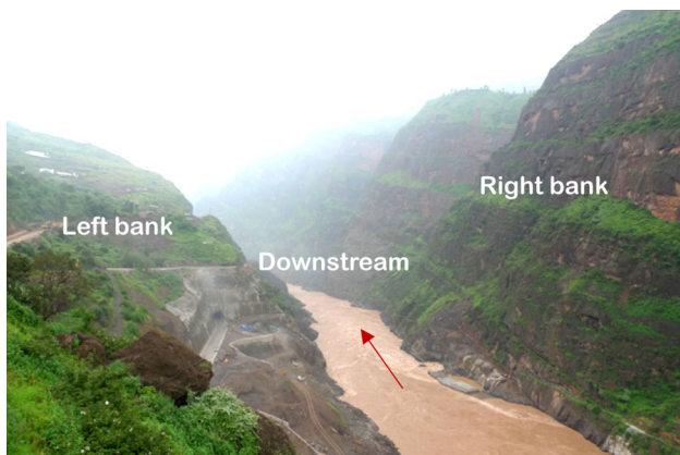
Fig. 2 Panoramic photograph of the Baihetan dam site: the slope of the left bank low and gentle, and the right bank slope is high and steep
