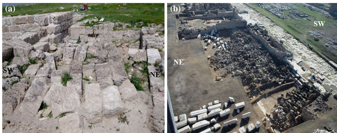
Fig. 12 Collapsed walls in Laodikeia antique city after the early seventh century AD earthquake. a Laodikeia Temple, b the North (Holy) Agora South Portik
