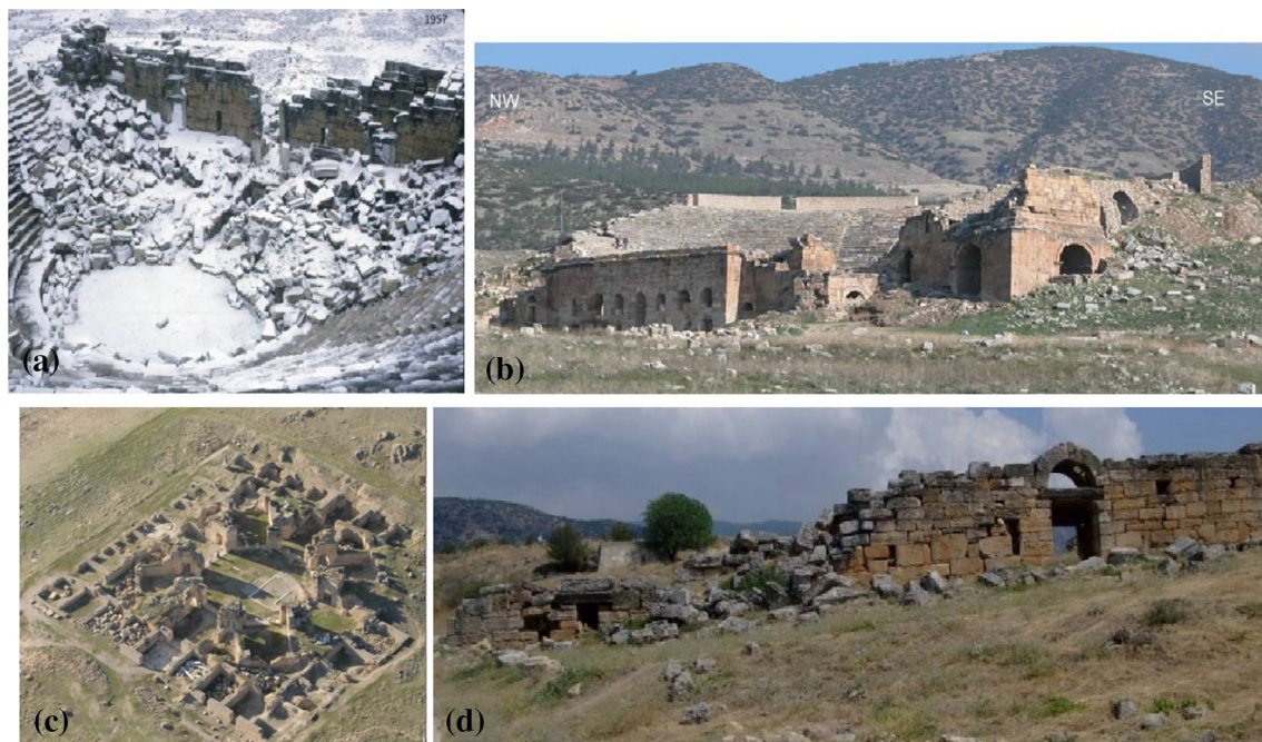
Fig. 8 a, b Damages at the great theatre of Hierapolis after historical earthquakes (location 7) (from Pamukkale 2009), c collapsed view of St. Philip's Martyrium built in early fifth century AD, d damaged part of the city wall at location 9
