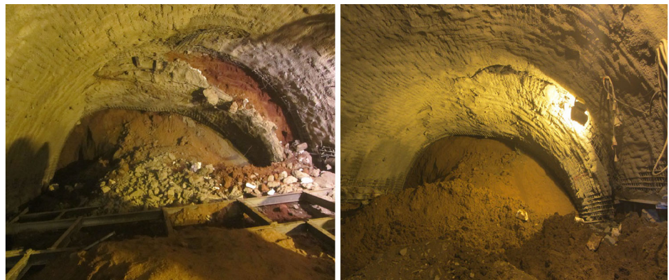
Fig. 6 Plastic zone around the tunnel without the pre-support system
