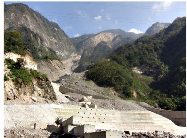
(b) Large deposits of debris remain over the Wenjia gully
