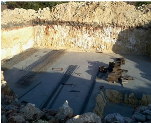
Fig. 5 Foundation level filled with concrete (view from E block foundation)
