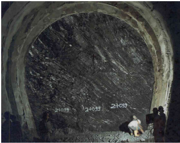
Fig. 2 Typical tunnel section showing the schistose and sheared rock mass
