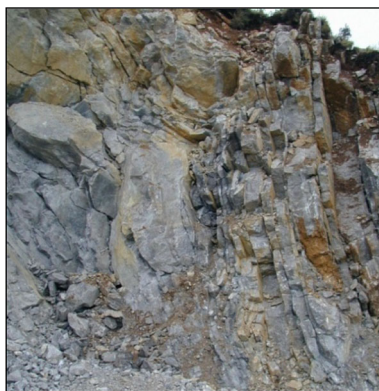
Fig. 15 Fault zone aspect
