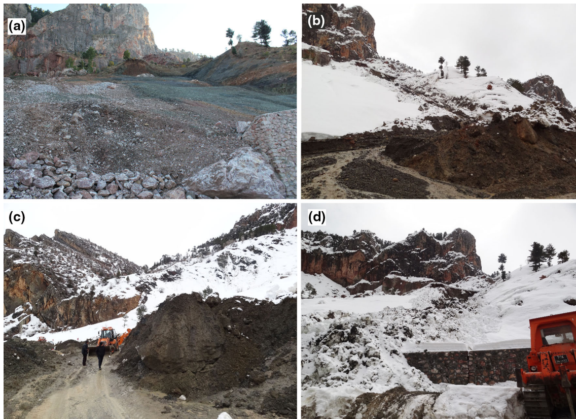
Fig. 3 a Result of floating work conducted by TCK during autumn months b landslide area and the earth that slid as a result of heavy snowfall c the large mass that slid d road-opening work done by bulldozers
