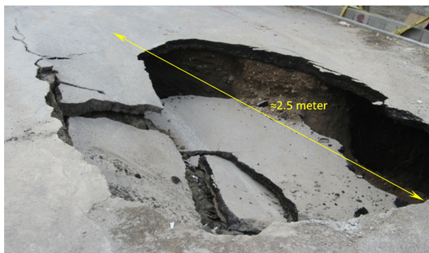
Fig. 7 Tunnel face instability and ground collapse
