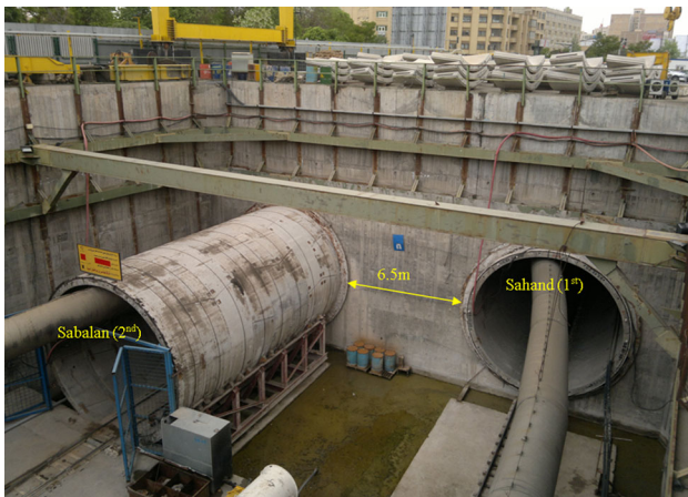
Fig. 18 Tabriz metro line 1 twin tunnels
