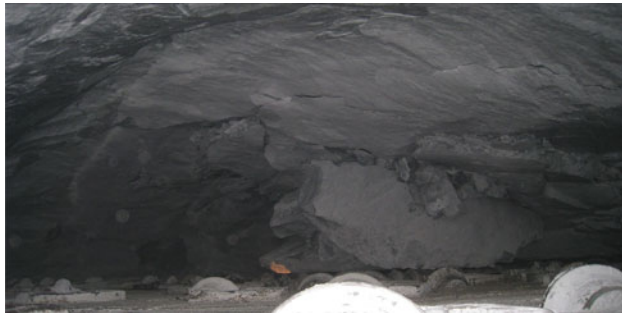
Fig. 8 Large block (2 × 2 × 4 m) ahead of cutterhead
