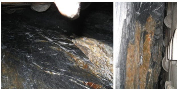
Fig. 5 Tunnel face at CH.15161.03 m in headrace tunnel 3 (medium layer rock mass)
