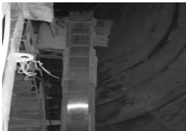
Fig. 16 Accessorial belt conveyor machine installed in TBM of headrace tunnel 1
