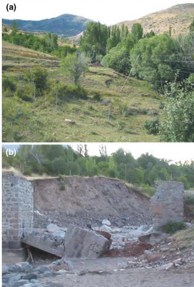
Fig. 2 a A view from landslides, and b bridge destroyed by Avutmus creek
