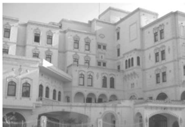
Fig. 3 A cladding application on reinforced concrete
