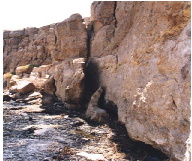
Fig. 3 Photograph showing the spacing of the joints and width of the fractures in the stronger strata located in the Wadi Ain Mousa area
