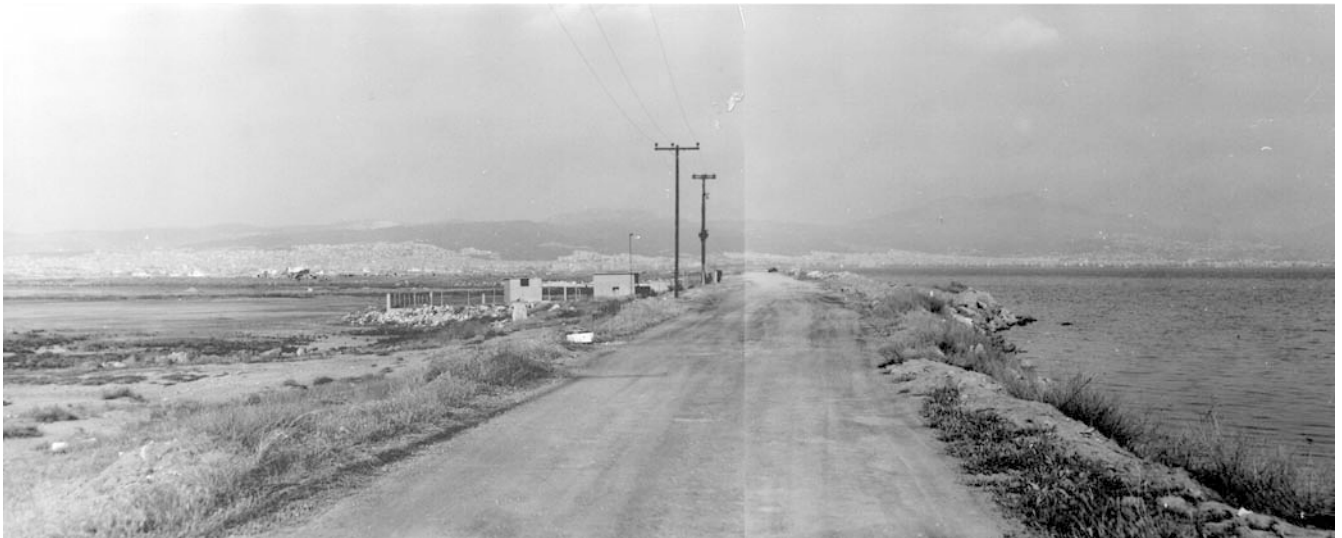
Fig. 5 Embankment along the coast at Kalohori village showing the pumping stations inland of the embankment
