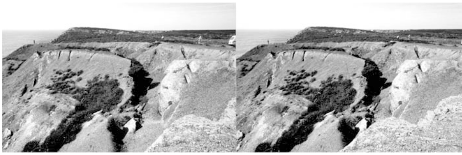
Fig. 11 Stereoscopic view (SSE to NNW) of upper part of the slipped block at Arrifana site
