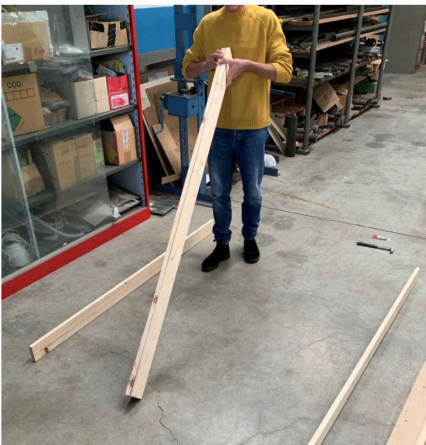
Fig. 11 Correct execution of the crowning operation
