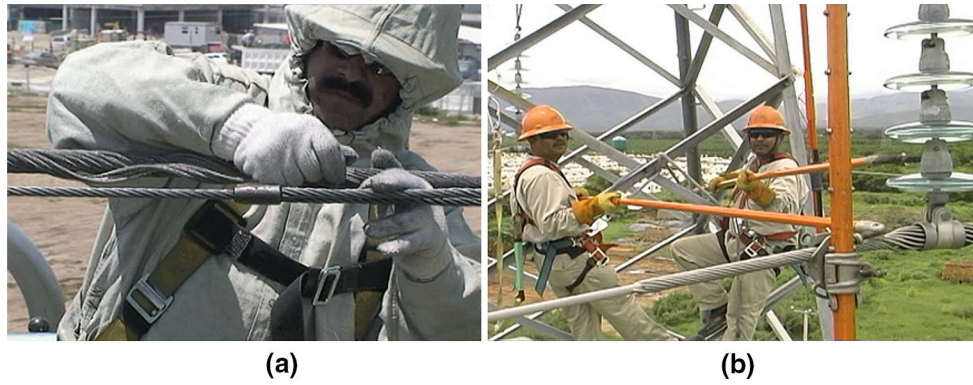
Fig. 2 Different maintenance techniques: a bare hand technique and b hot stick technique
