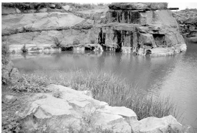
Fig. 3 Photograph shows the sheet joints in the granite basement rock in the exposed quarry near Hyderabad, which act as potential groundwater zones
