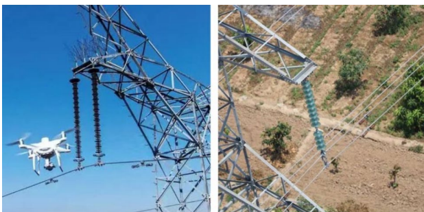
Fig. 1 The UAV inspection process (left) and the self-exploding insulator photographed by a UAV (right)
