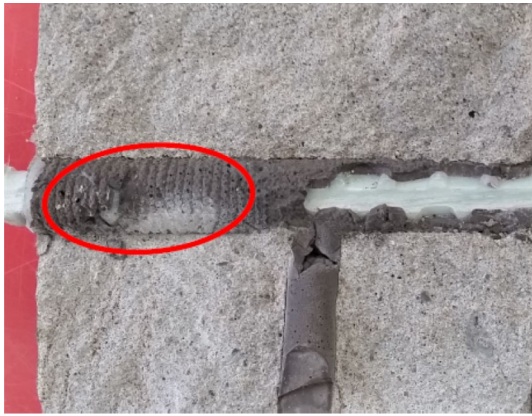
Fig. 10 Grouting quality examination after testing
