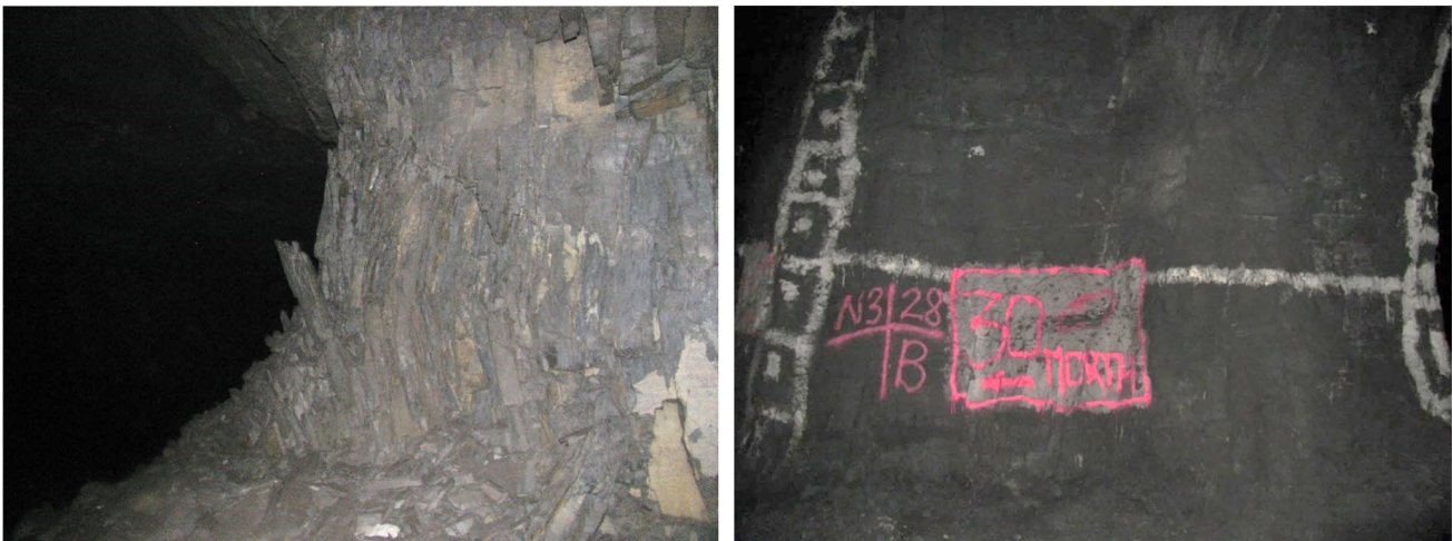
Fig. 2 Different manganese pillar behaviours caused by the number of joint sets and the spacing of the joints
