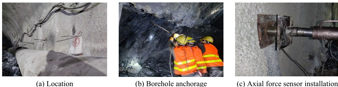
Fig. 21 Stages of the construction process
