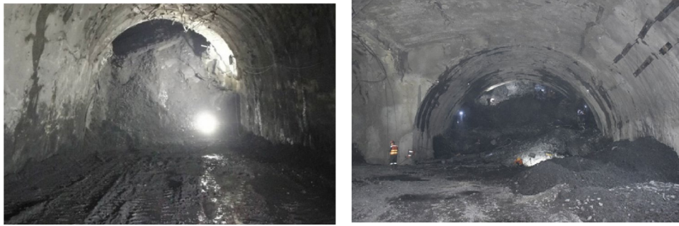
(a) Treatment effect of asymmetric large deformation disaster
