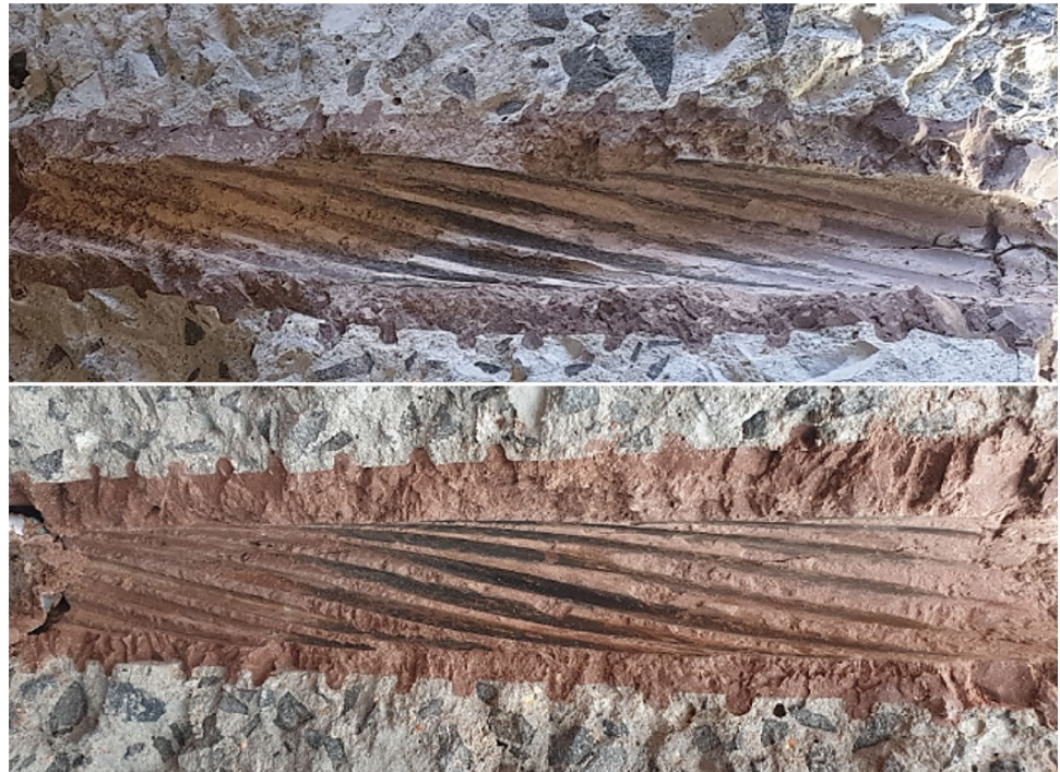
Fig. 21 Top: opened 12 strand cable with rotation allowed, and bottom: opened 12 strand sample with restricted rotation—borehole collar on right
