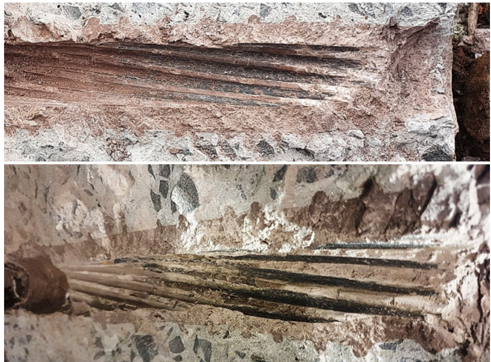
Fig. 22 Top: grout condition after 10-strand test with 60 Nm torque, and bottom: grout condition after 10-strand cable test with 80 Nm torque—collar on the right
