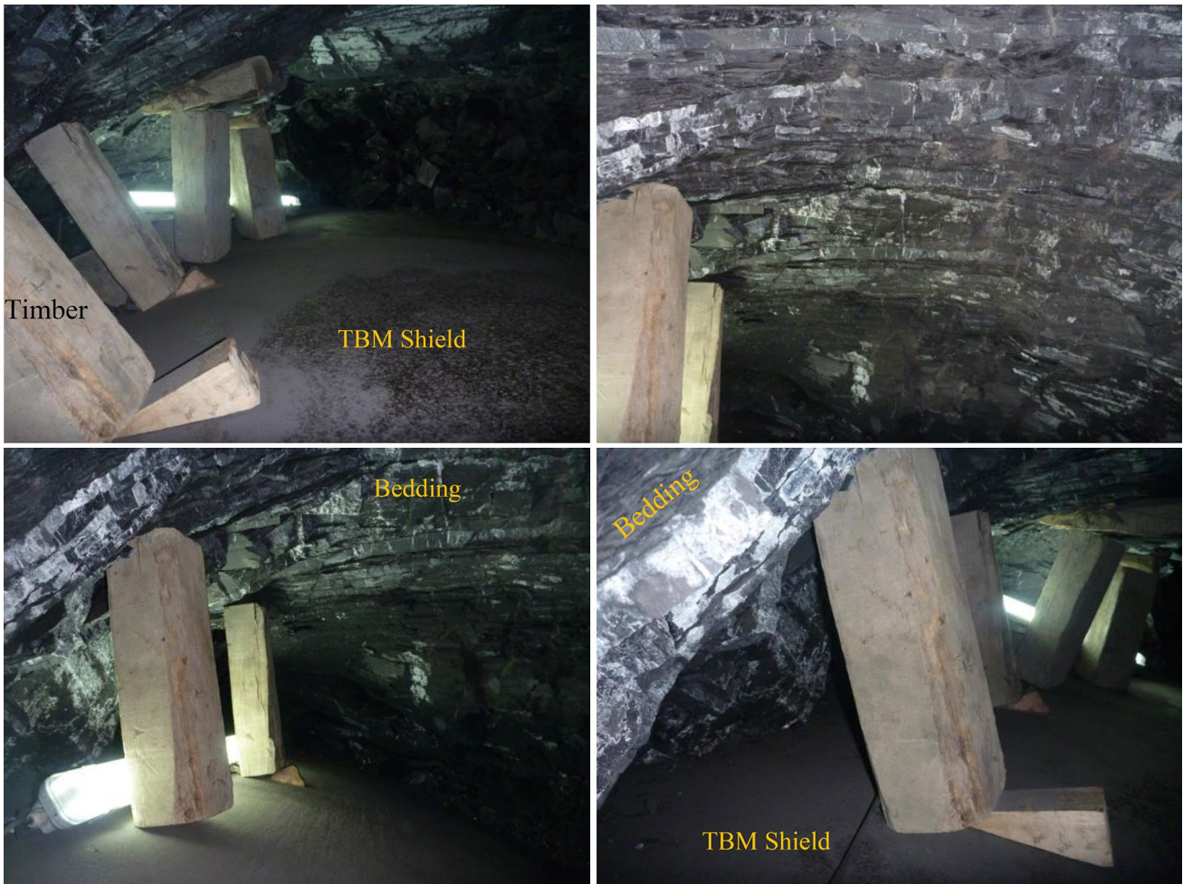
Fig. 24 Timbers used to facilitate the TBM releasing operation
