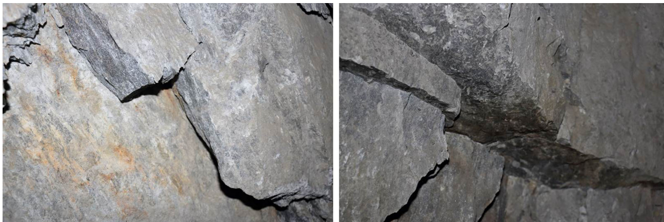
Fig. 3 Example of joints observed on the surface of exposed dyke on 3710 Level
