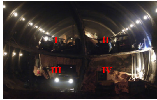
Fig. 15 CRD excavation
