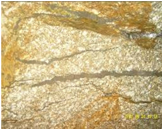
Fig. 14 Rock surface after grouting
