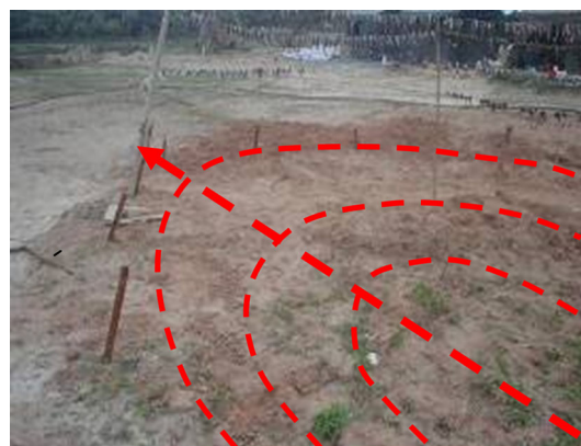
Fig. 22 Ground settlement trough
