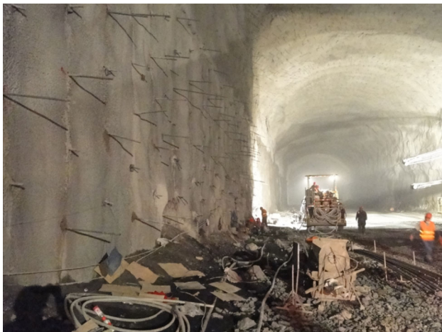
Fig. 22 Stability of tunnel sidewall at chainage K0 + 300 to K1 + 350 at No. 3 diversion tunnel with support parameters designed by the cracking restraint method
