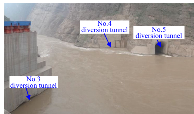
Fig. 33 Diversion tunnels under safe operation
