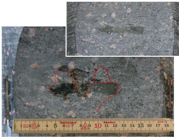
Fig. 13 Front view of the spalling area at side 1 on KS0044B02. Chips have fallen off in the darker areas (cf. small photo of the same area before testing). The holes after the missing rock are like small craters. The extent of the fractures is marked with red lines (about 75 mm × 45 mm)
