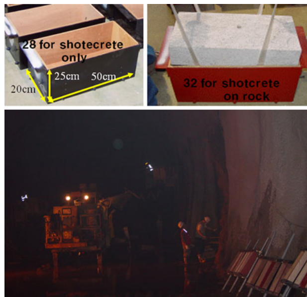
Fig. 2 Mold preparation and placement in a tunnel
