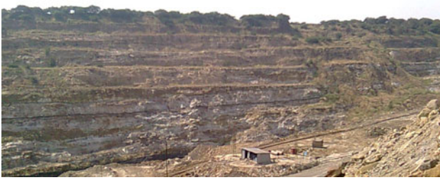
Fig. 2 Dip side slope of NKOC mine showing the localized instabilities
